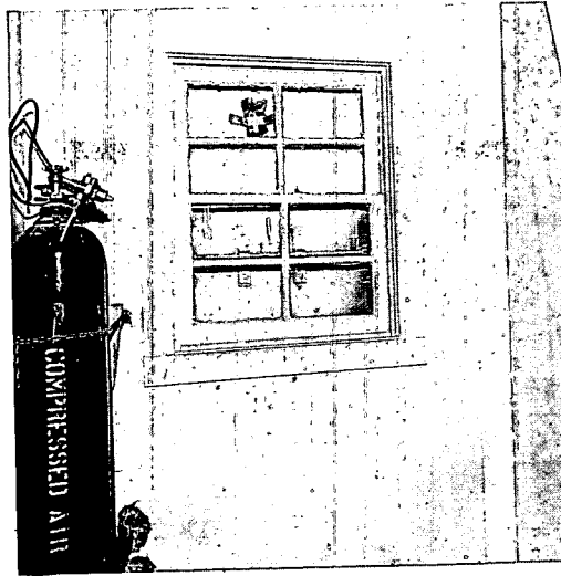
Fig. 9—Interior of concrete bathroom shelter showing window detail.
